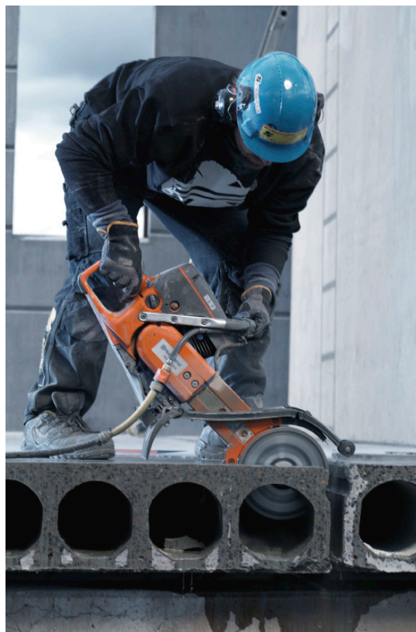
Efficient. With the new Husqvarna deep cutter, you easily cut in stages through walls of up to 400 mm thick. .
